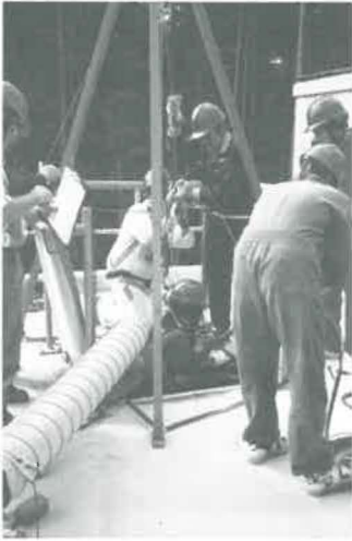
The above ground team lowers a rescuer into the confined space.
