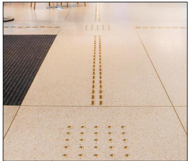
Figure A7: Use of Colour-Contrast and Tactile Direction Indicators on Flooring
