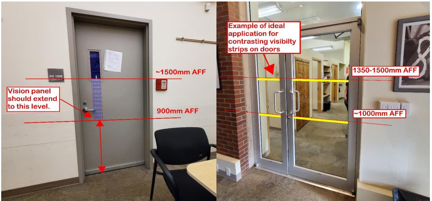
Figure 3.3 – Inaccessible glazed door panels
