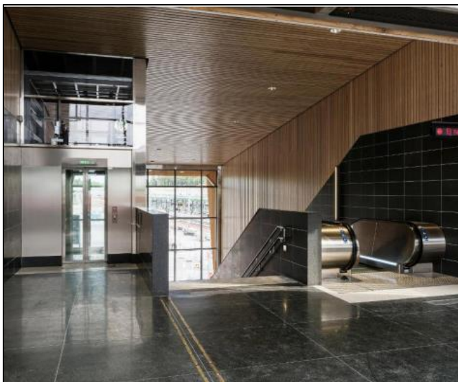
Figure A7: Use of Colour-Contrast and Tactile Direction Indicators on Flooring
